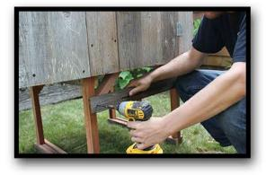
Final Step: Attach your Ladder Bar 3-4 inches below the opening of your Front Door. This will be a resting spot for your Ladder. Make sure you can open and close the Front Door. (Note:: If you are buying a Run, this step will not be necessary, as your Ladder will stay inside the Run.)
