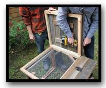
Step Three: Turn the Bottom Frame over so that it will act as a table. Proceed to use your screws to attach the Frontside (Door) and Backside Panels to the bottom frame. These panels will be on opposite sides of the coop. Make sure that the nesting box (the side with two floor planks) is on the left of the front door, as is pictured.
