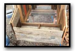
Step Seven: Next, install the Nesting Box Hinged Door. Make sure it is flush, and secure it to the Bottom Frame. Once secured, you can also screw the Nesting Box Dividers into place.
