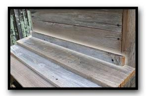
Step Eleven: Place and attach the Nesting Box Weather Strip on top of the Nesting Box Roof so that its 18° slanted edge allows it to fit snugly against the roof and side-walls. This Weather Strip will help to seal your Hen House from the elements. Additionally, you can apply liquid nail to seal any gaps.
