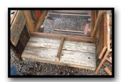
Step Six: Install the Long Nesting Box Divider by nestling it between the two Side Panels. The Short Nesting Box Divider will lie perpendicular, midway. (As shown to the left.)
