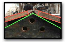
Step Thirteen: Place the Roof Panels, and double check the ridge line. Make sure it is even across both the front and back sides of the Hen House.
