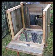
Step Five: Slip the Nesting Box Sides inside the Front and Back Side Panels. Be sure to check that they are level with the bottom boards and screw them into both the Side panels and the Bottom Frame.
