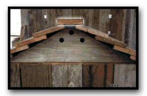
Step Fifteen: To complete the Hen House, find the Center Roof Cap and align it evenly across the two Roof Panels. Place 4 screws evenly across the ridge into the attached roof panels.
