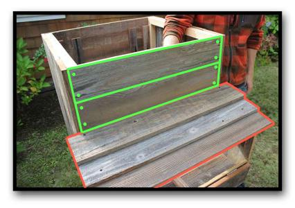
Ensure that the Nesting Box Roof (outlined in orange) is centered before you attach it, so that it hangs off of each side equally.
